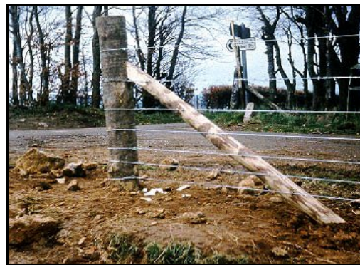
Figure 10.1 Conventional Strainer Post
