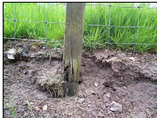
Figure 10.6 Base of Fence Post Rotting at Ground Level
