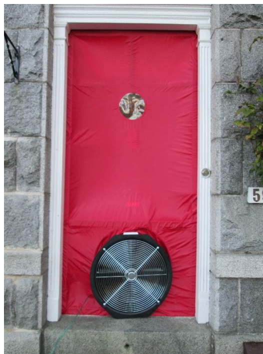
Figure 6.1 Pressure test kit installed in front door of house
