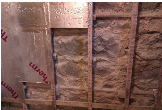
Figure 5.1 Sheets of 50-25 mm insulation fixed between studs with foil tape, leaving 50mm air space between sheet and wall
